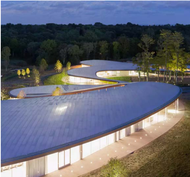
‘Close to sublime’ ... the five glass pods glow beneath the rooftop by night. Photograph: Iwan Baan/Grace Farms
